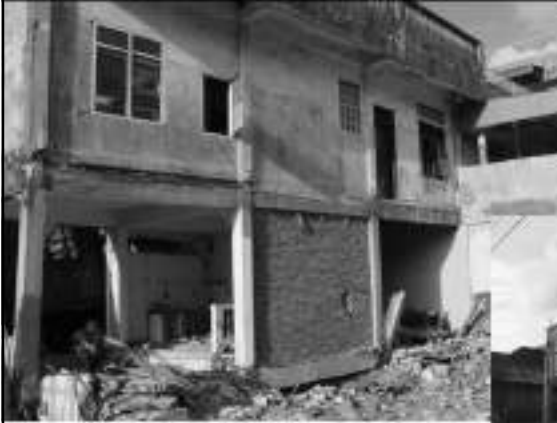
Soft story of typical commercial buildings - failure of 1 st story
