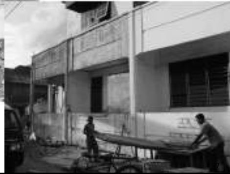
Soft story of typical commercial buildings - failure of 1 st story
